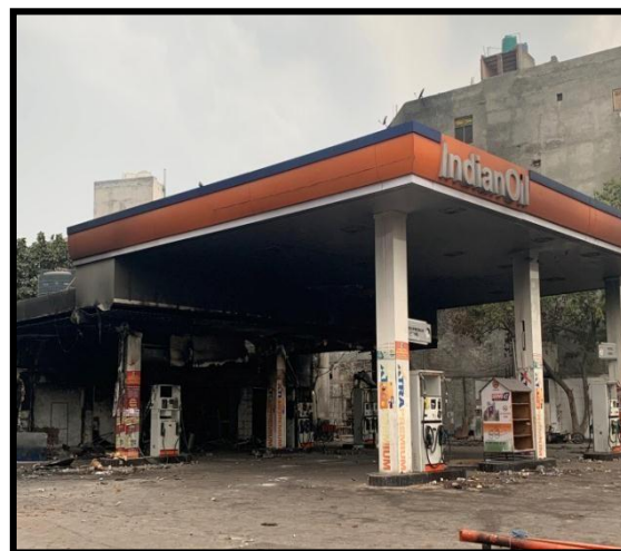
Burnt Petrol pump of Bhajanpura
