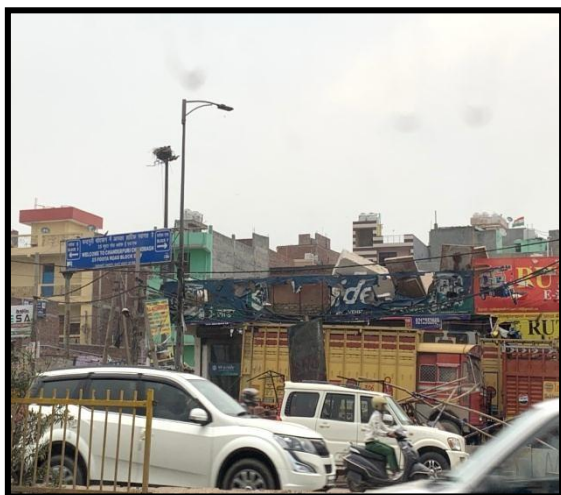
Road across burnt Bhajanpura petrol pump
